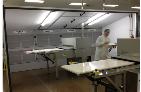
Vertex booth, eight modules in use.
